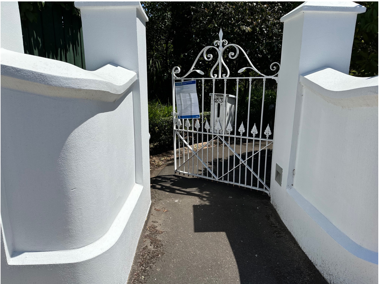
Photo showing Interim Protection Order on front gate of Halstead (Photo GEHS March 2025)
